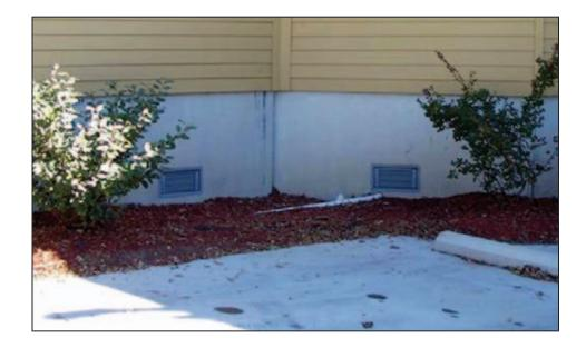
Figure 6-43. Example of flood vents
