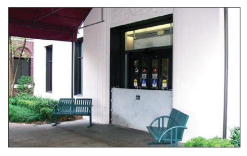
Figure 6-41. Example of a flood shield over a door
